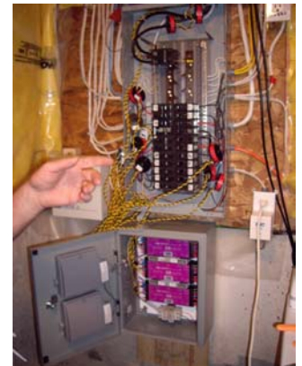
Electrical Sub-metering
