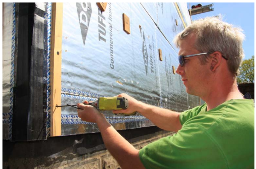
Home Energy Retrofit
