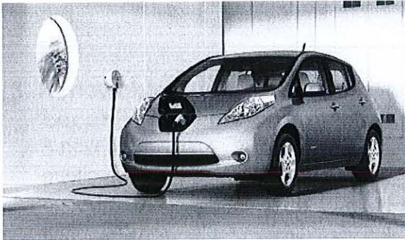
Electric Vehicle Charging
