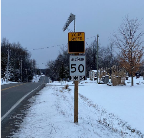
Westbound 57 East of Williams Point – Radar Feedback Sign
