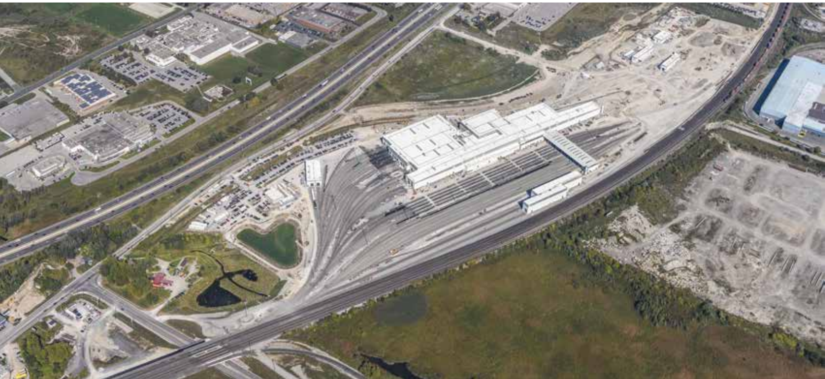
New GO Rail Maintenance Facility in Whitby. Notice the white roofs and white walls. Photo courtesy of Town of Whitby and Metrolinx.
