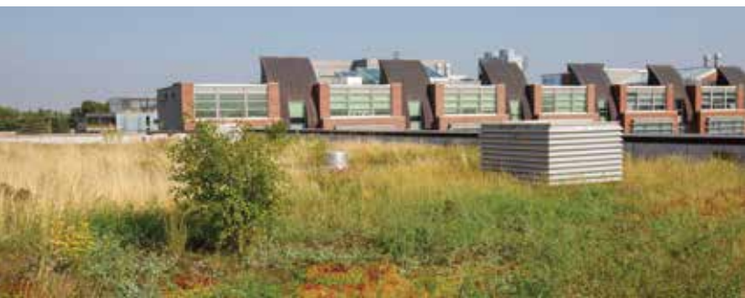
University of Ontario Institute of Technology green roof. Photo courtesy of Calvin Taylor/UOIT
